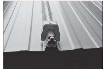
Example of correctly installed S-5-KHD clamp
